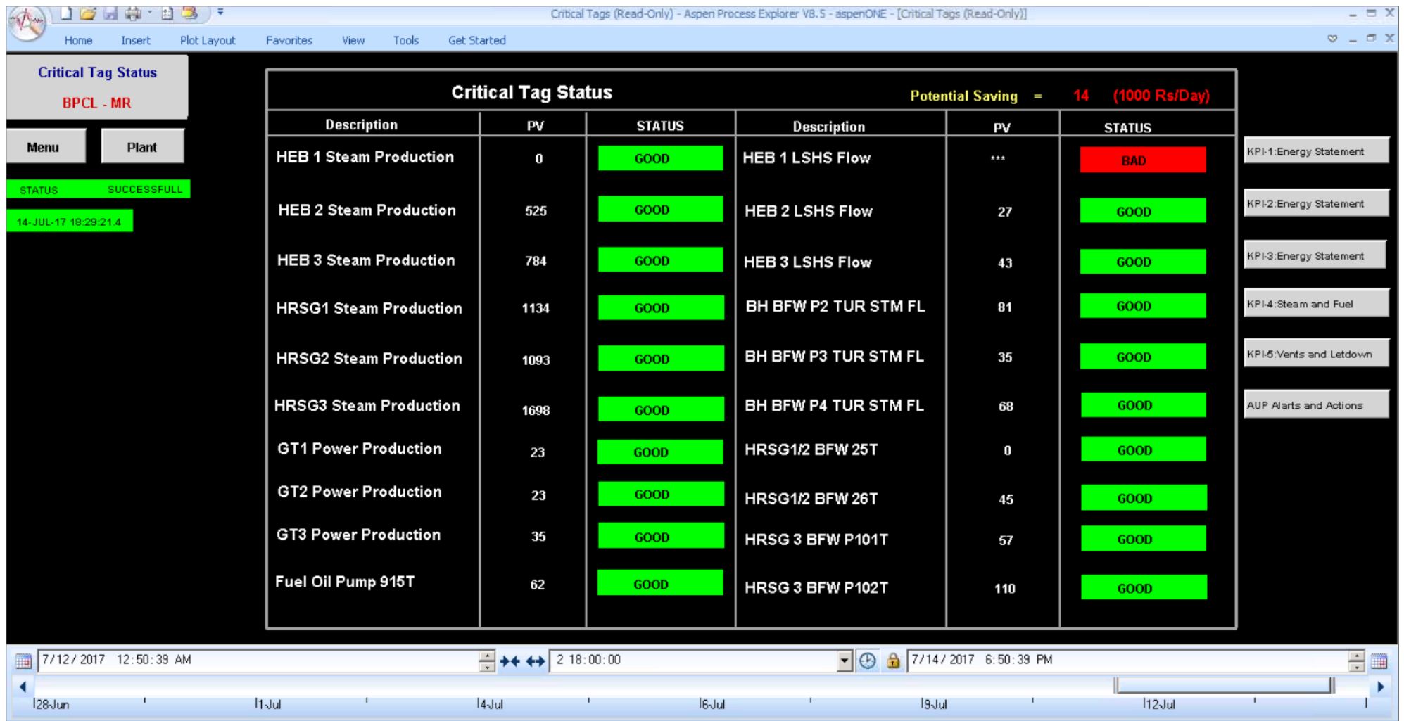
Figure 9: Critical Tag/Meter Status
